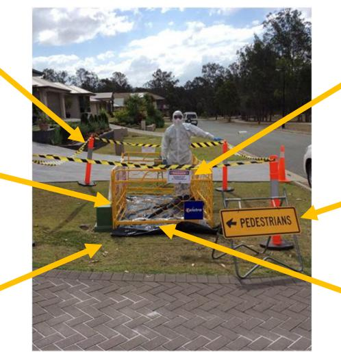
SIGNAGE Set up 2 'Danger Asbestos Removal' signs on the Asbestos Work Area (one facing each direction of traffic flow)
