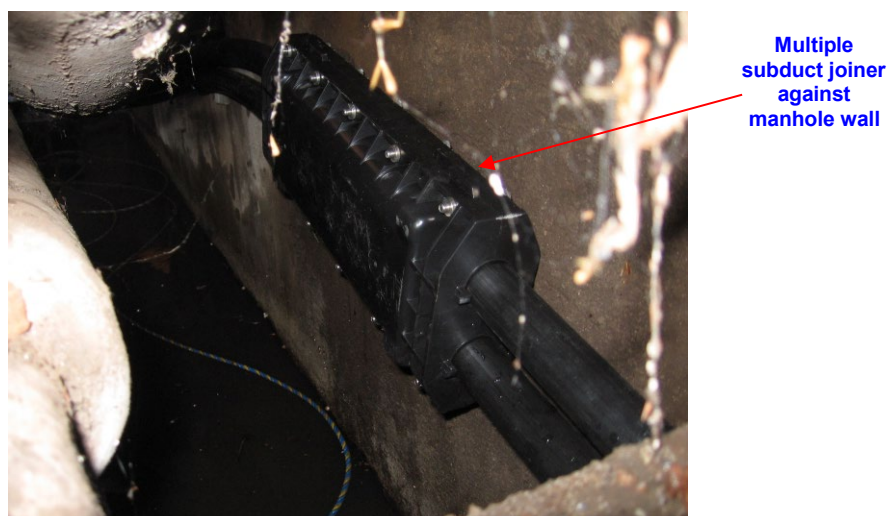
Figure 7 – Typical Installed Multi Subduct joiner
