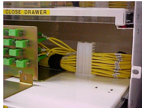
Figure 6 - Pigtails Labelled at rear of Patch Panel
