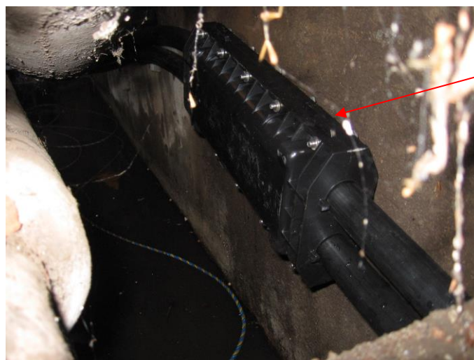
Figure 7 – Typical Installed Multi Subduct joiner
