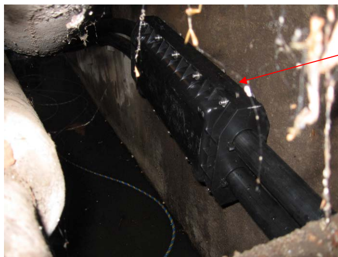
Figure 7 – Typical Installed Multi Subduct joiner
