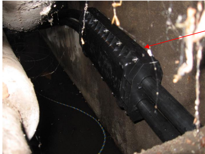
Figure 7 – Typical Installed Multi Subduct joiner
